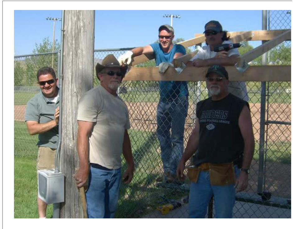
Above: Volunteers rebuilding a dugout at Meadowbrook Park (TVRPD Facebook page)
